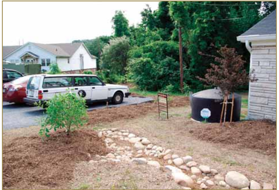
Upper Etowah River Alliance Low Impact Development (LID) Education and Demonstration Facility. Below: Compost filter sock used to filter stormwater before discharge into endangered species habitat section of the Etowah River.
