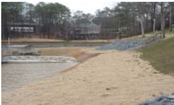
Shoreline After Restoration
