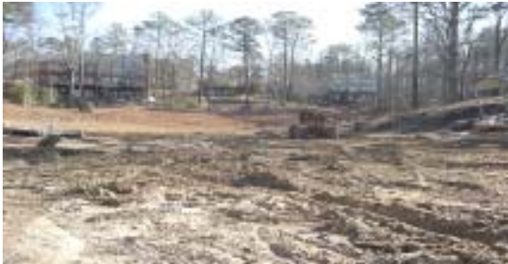
Shoreline Before Restoration
